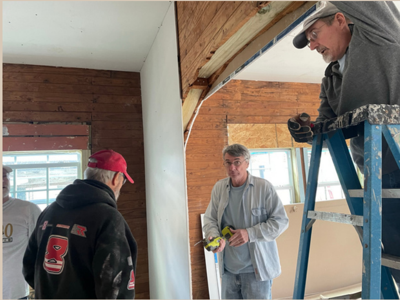
SCOTT, JEFF, AND STEVE HANGING DRYWALL
