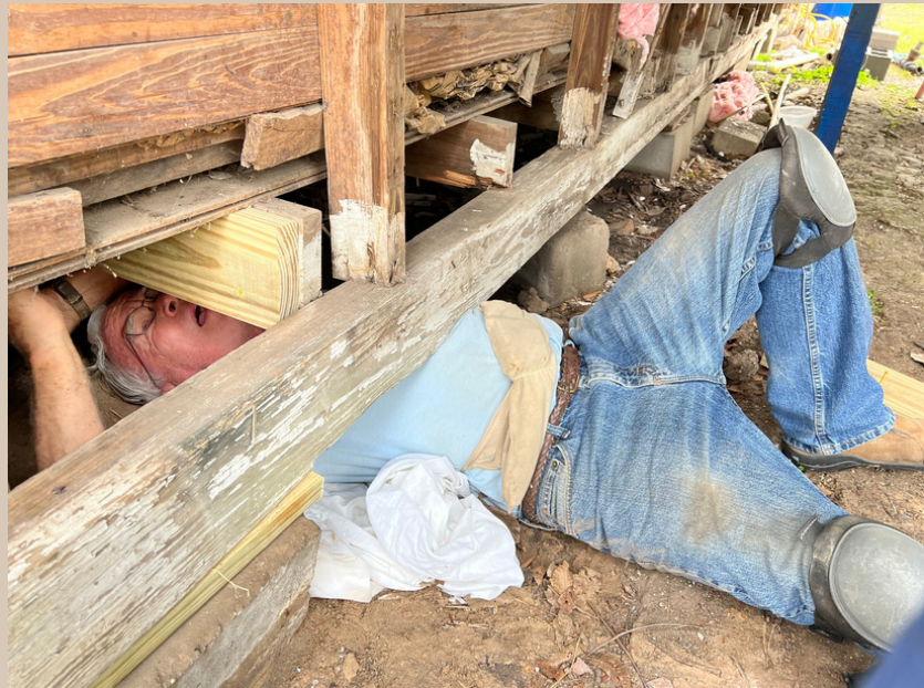
EARLY GETTING DIRTY REPAIRING THE FOUNDATION
