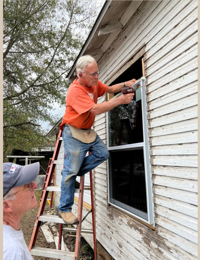
EARLY INSTALLING A NEW WINDOW
