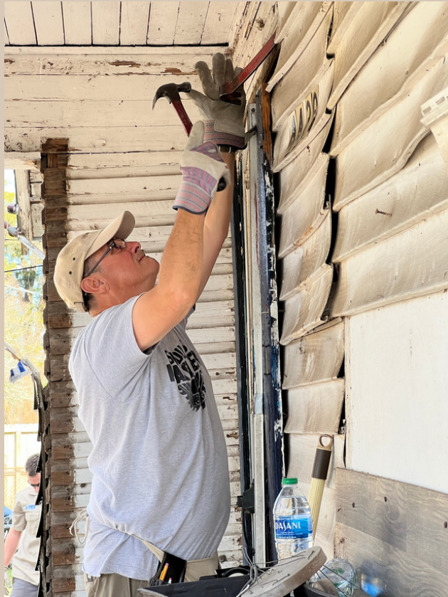
JOE REPAIRING SIDING
