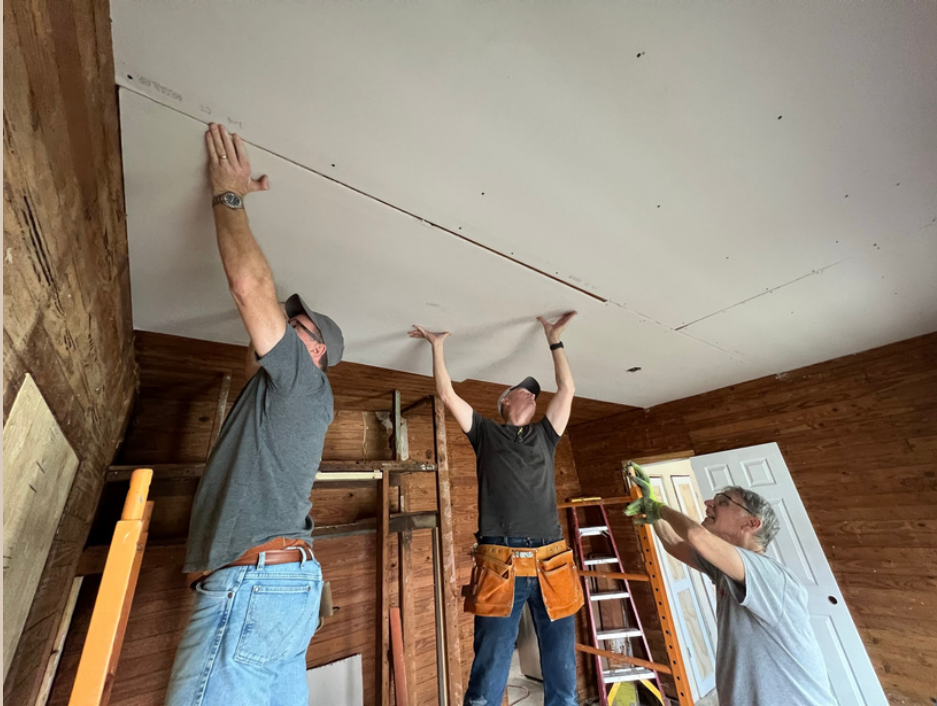
DAVE, JIM, AND ROBERT HANGING CEILING DRYWALL (DAVE SUPERVISING)
