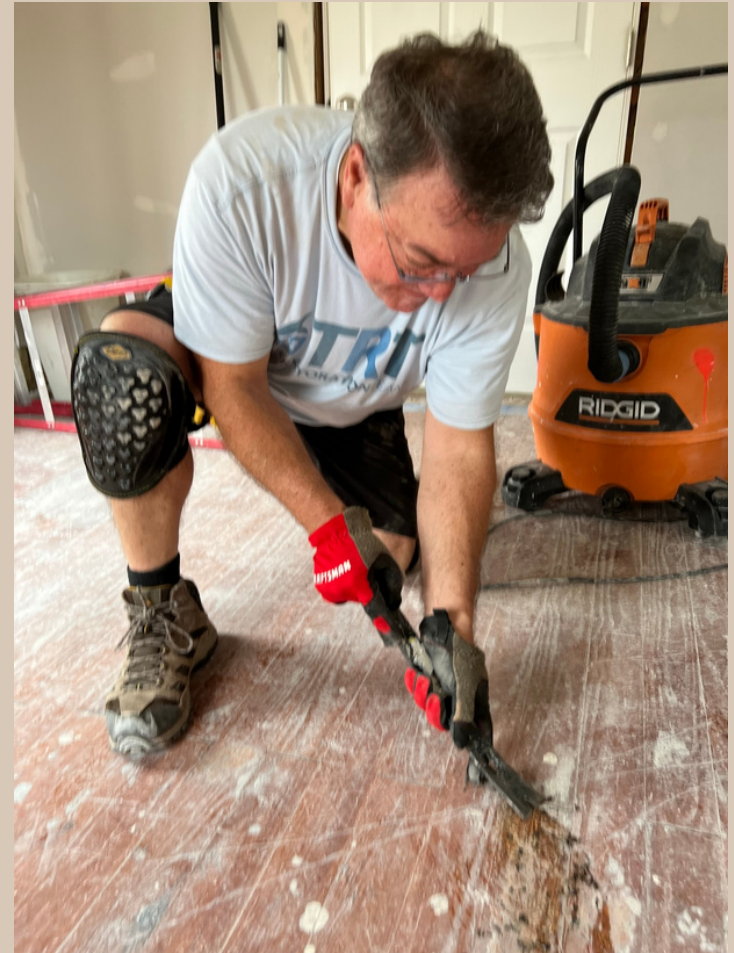
BOBBY REPAIRING FLOORS
