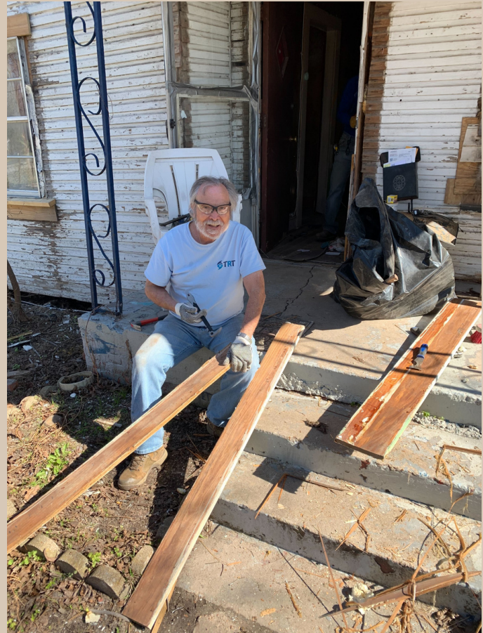
SCOTT PULLING NAILS OUT OF BOARDS
