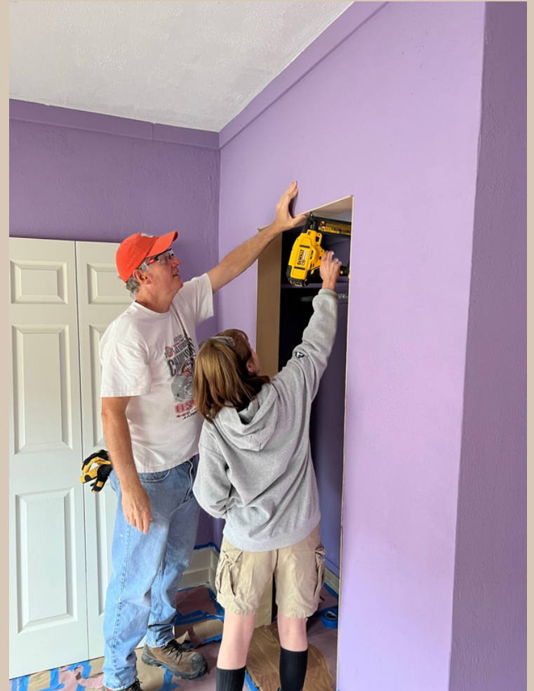
DAVE AND MORIAH INSTALLING A NEW DOOR
