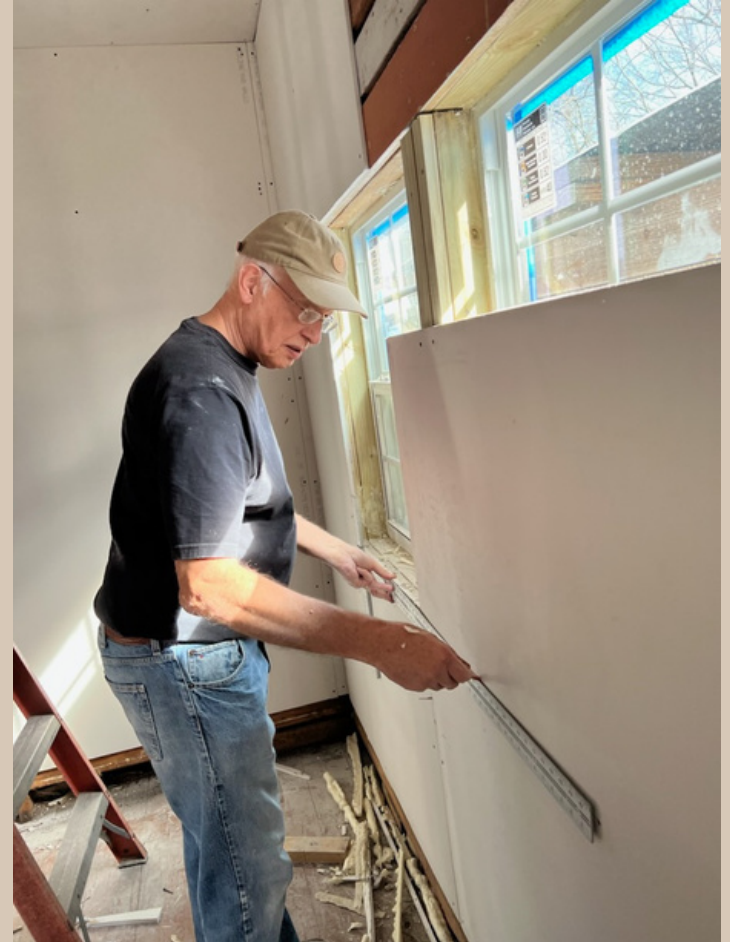
PHIL HANGING DRYWALL
